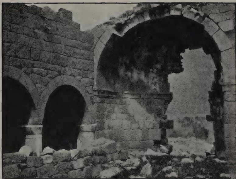
FIG. 19.—No. 4, interior of apse.
